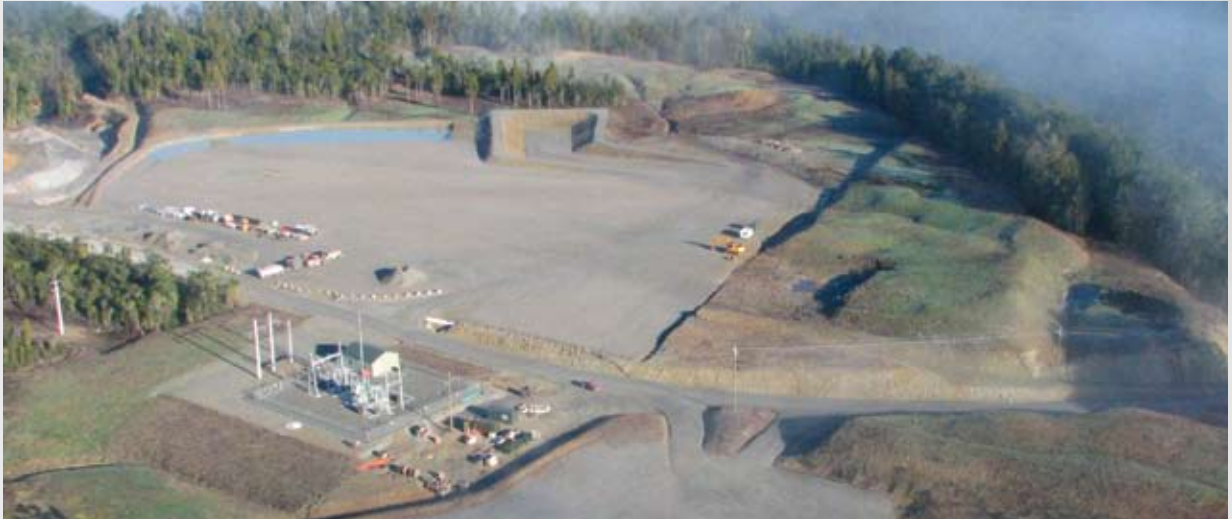
Aerial view of the coal preparation plant area
