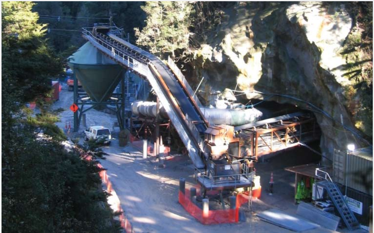
Conveyor removing rock from tunnel
