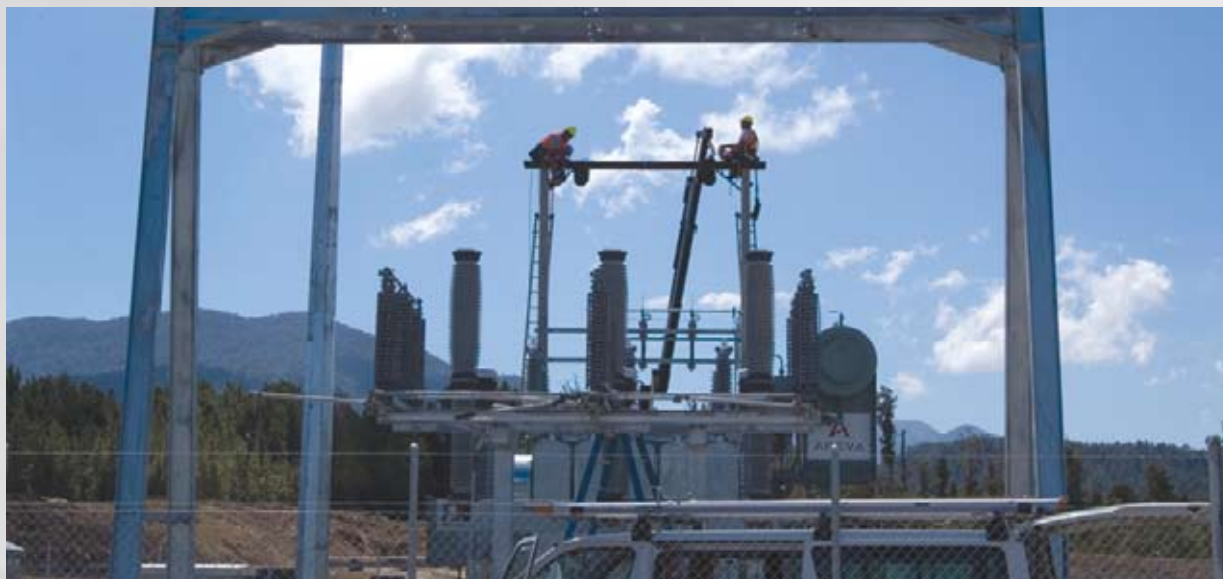
Electricity infrastructure being installed
