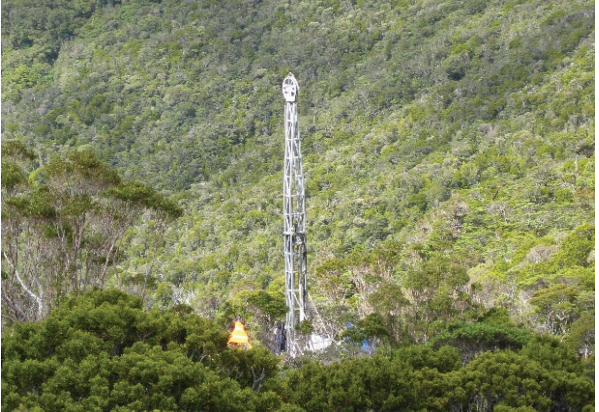
Small drill site with rig installed by helicopter
