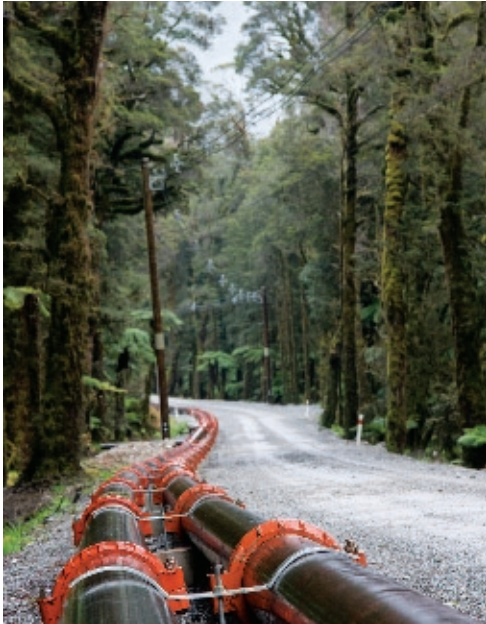
Coal slurry pipeline winding through trees
