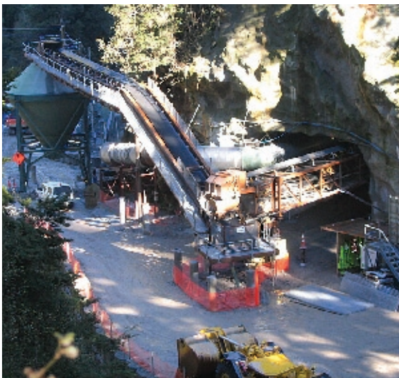
Mine portal entrance into the Paparoa ranges
