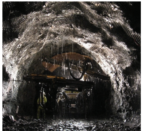
Access tunnel under construction
